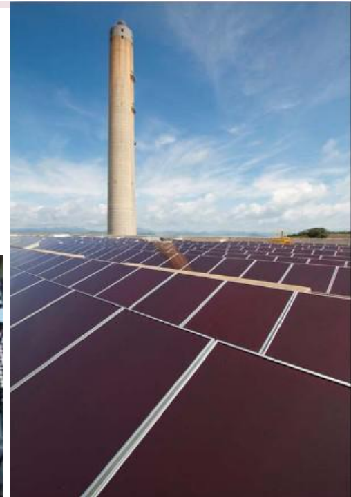
Lamma Power Plant
