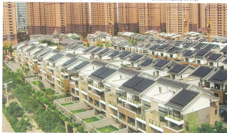
The household solar project of Shoufu Villa in Hualbei of Anhui (Installed capacity: 264 kWp)
